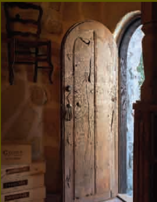
Arched wine cellar entry. Constructed with antique mesquite panel and reclaimed Douglas Fir. Features antique clavos and strapping and reproduction hardware.
